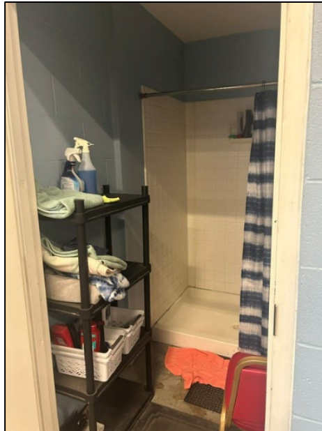
Crew Shower Stall in Apparatus Bay
