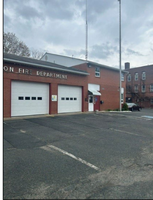
Partial View of Front Pad (west side of the building)
