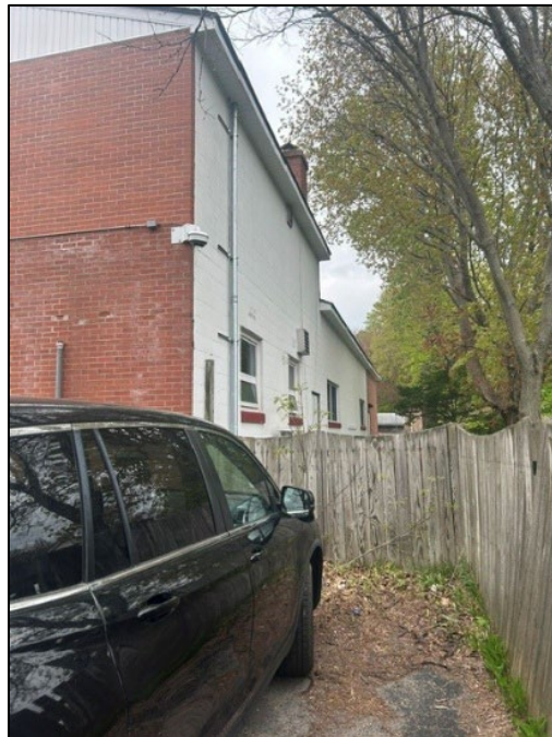
Rear of Building at Charlie/Delta Corner (east side of the building)
