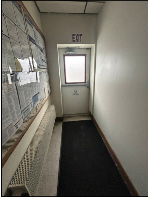
Exit Corridor – 1 st Floor
