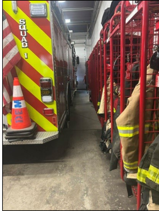
Close Clearance of PPE Racks to Apparatus
