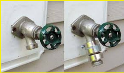
HOSE BIB VACUUM BREAKER BREAKER
